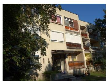
**Figure 1**. Some households in this block suffered from overheating, while others did not – it depended on whether they had external blinds and/or were shaded by the trees. The top floor had problems, but the middle floor pictured here had external blinds so did not face the same issues. (Photo by Neil Simcock)
